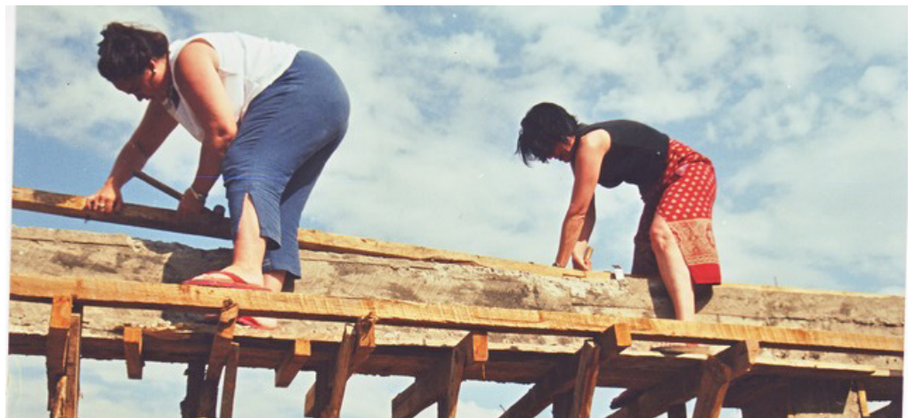
As our first two-storey buildin was being constructed, Kim and I quickly realised that the beams for the roof were lopsided, so we set about pulling them apart.
